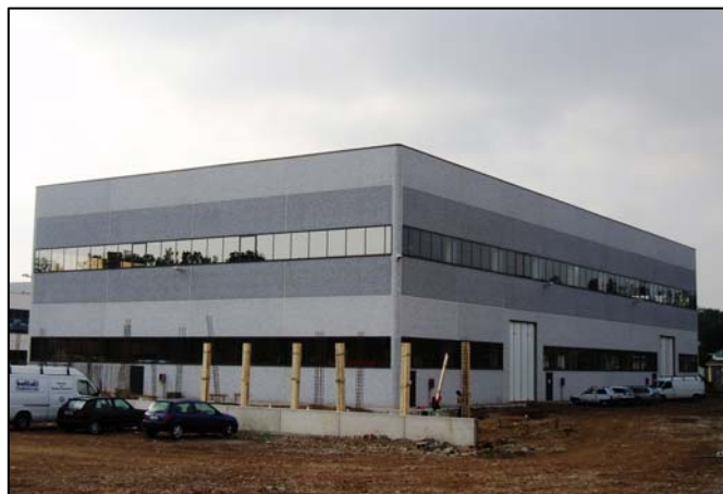
External view October 2005. Office construction ongoing.
