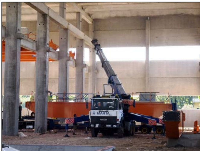
Bay #1 July 2005. Installation of the 100t crane.
